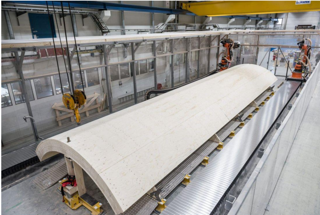
A wooden tower module being put together.
