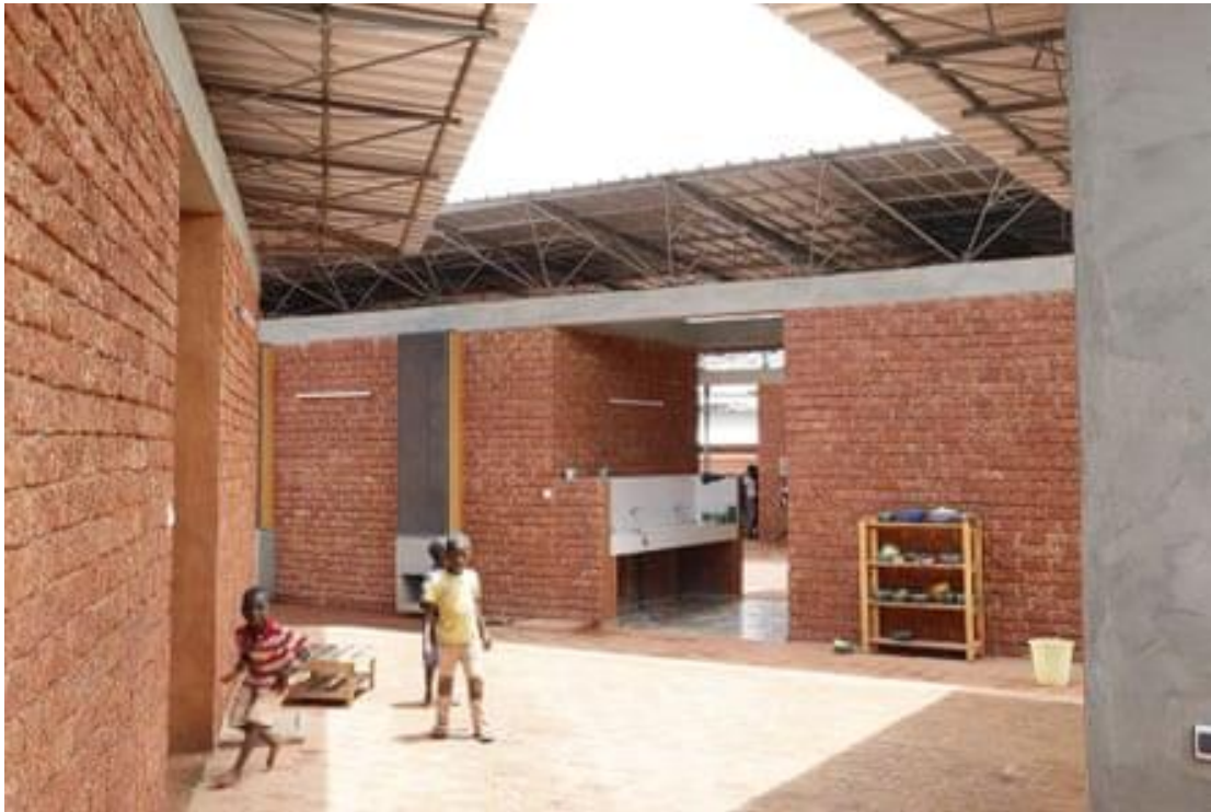
The Noomdo orphanage, where metal plates above the rooms protect them from direct sunlight and rain. Photograph: Iwan Baan/Kere Architecture
