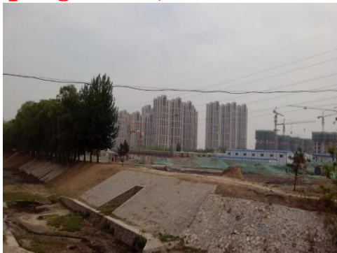
Before (concrete channel)
