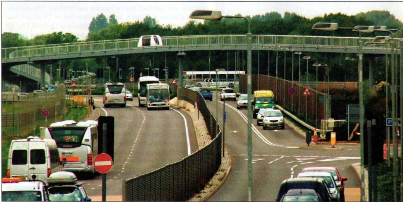
Figure 5. The low-profile guideway was built over two rivers and seven roads without requiring any highway or service diversions
