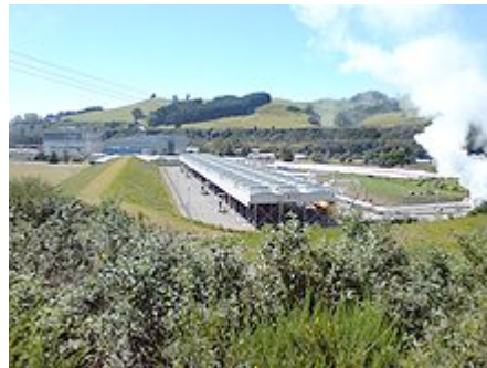
Figure 6: The Wairakei geothermal power station. The two main blocks are at the left rear and the binary plant is in front.
