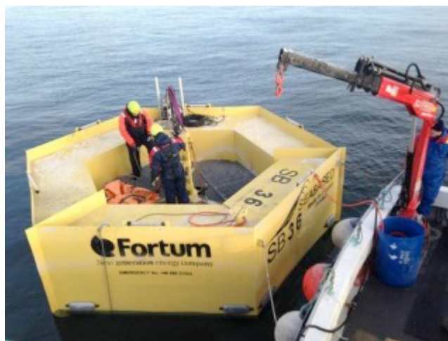
Figure 3: Buoy being attached at the Sotenäs wave energy plant. A cable running to a generator on the sea floor allows energy to be captured from waves. Attribution: Seabased.
