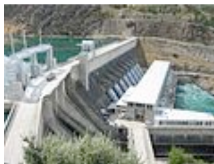
Figure 2: Roxborough hydro dam, Clutha River, showing the eight penstocks, generation capacity 320 MW. Attribution: Kelisi (CJMoss), Creative Commons
