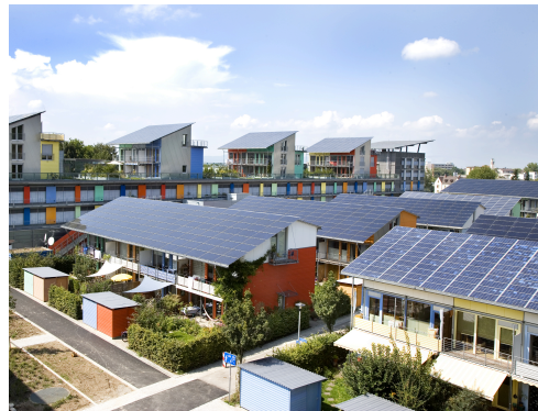
Figure 5: The Solar Settlement, a development of 59 homes in Freiburg, Germany, that produce more electricity than they use. Attribution: Andrewglaser at English Wikipedia
